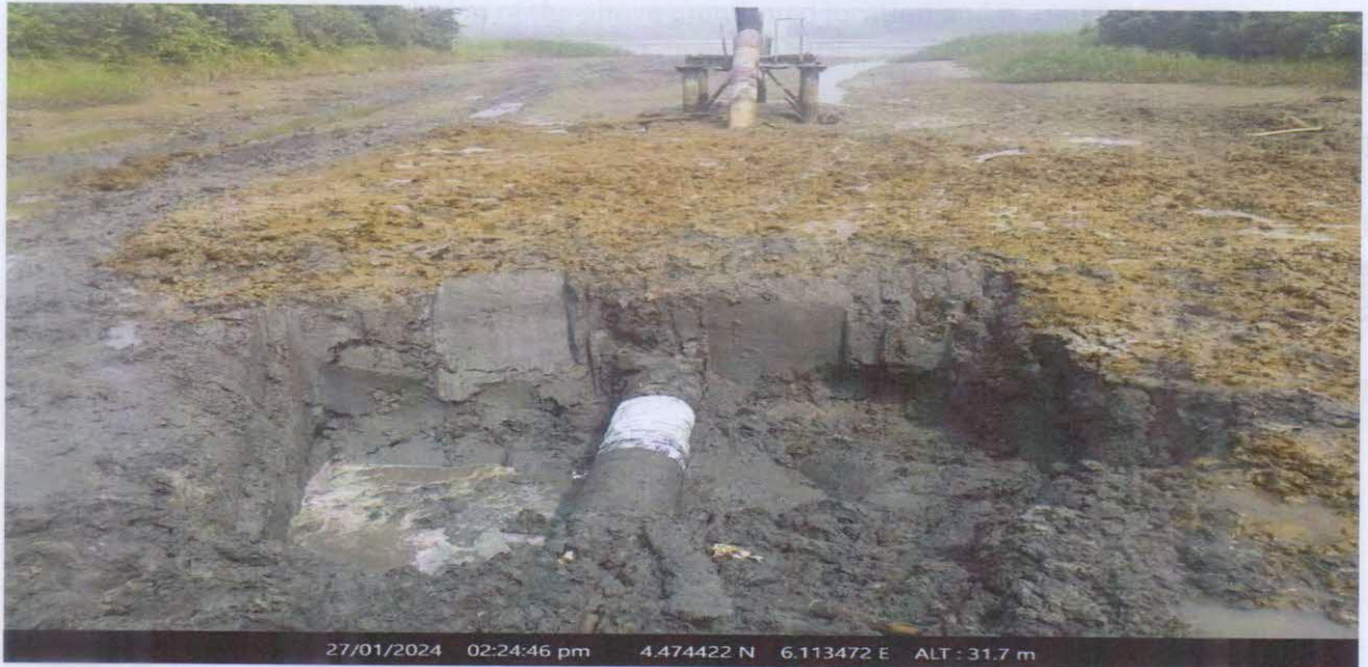
Repaired incident point
